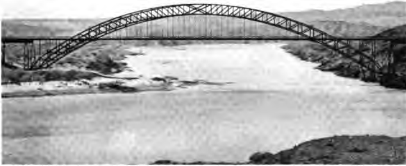
Looking down river at Colorado River bridge at Topoc, Arizona.
